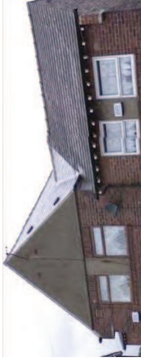
Typical detail of the overhanging eaves, brown/grey roof tiles, flat brick arches and specials as heads and cills to the windows, corbelled precast concrete and brick supports to the eaves and plastered gable top
